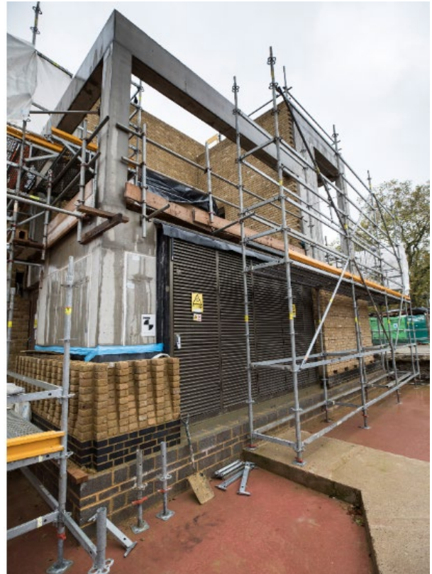
Figure 4 - Brickwork cladding on the headhouse
